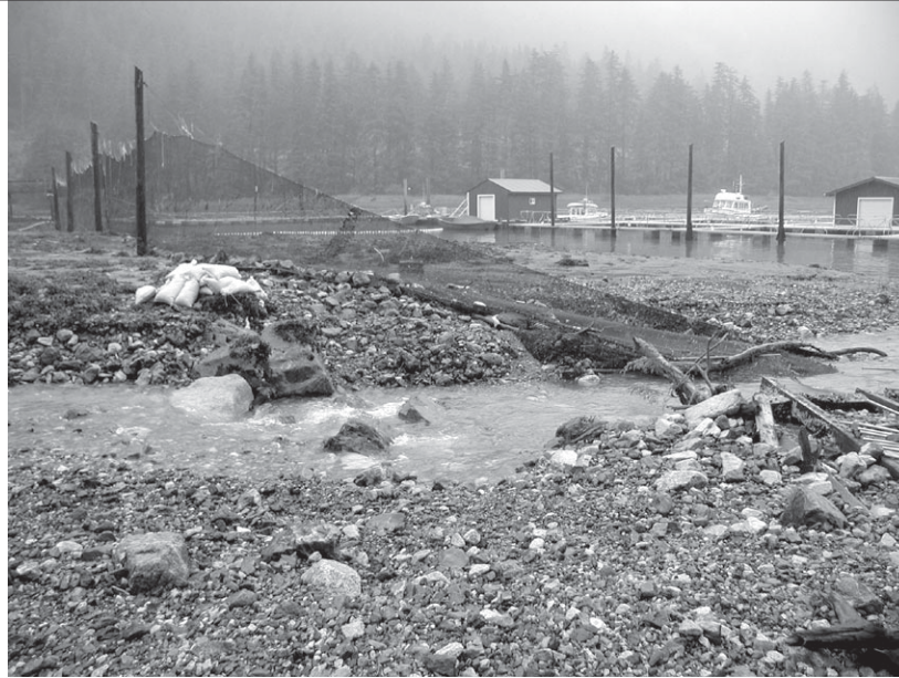
Remnants of the weir on Medvejie Creek lie buried in debris after an August storm just days prior to chum broodstock returning to Medvejie this year.
