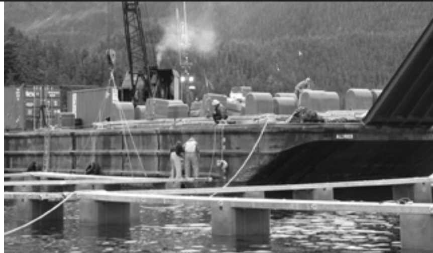
The Hidden Falls staff assembles net pens for the Takatz chum salmon program during September. The new net pens will be towed to Takatz Bay in March 2004 for the 45 million chum fry rearing program.
