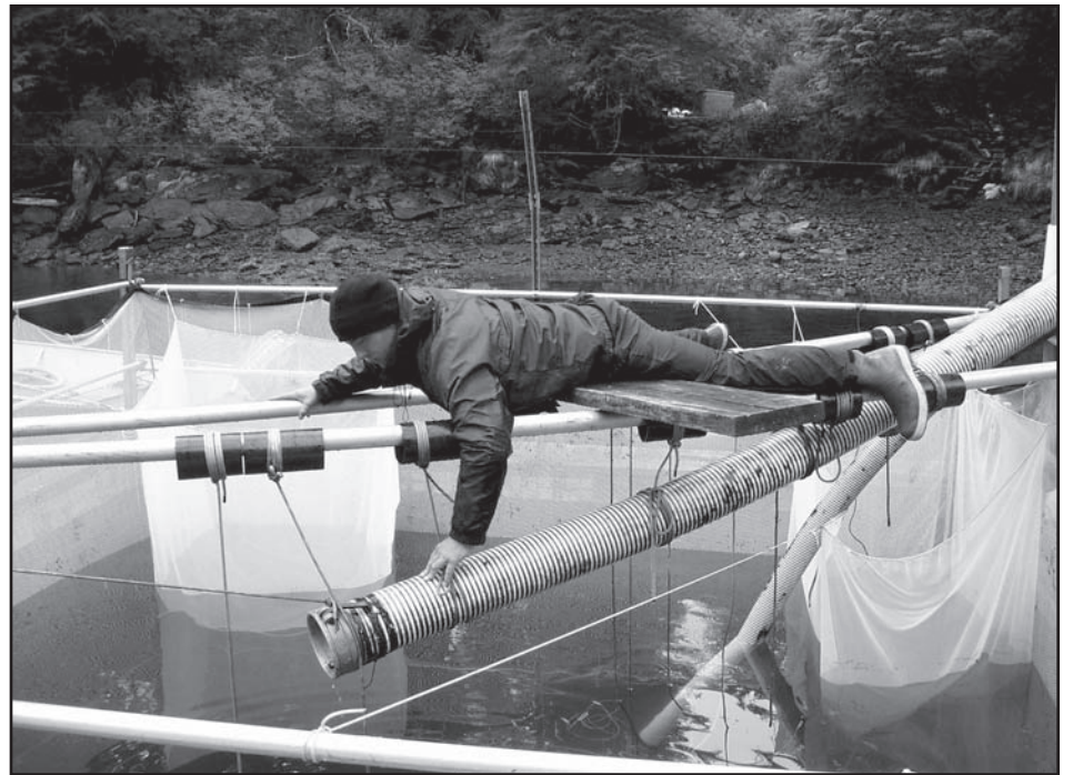
Installing the smolt pipeline at Mist Cove can sometimes be a balancing act as Tommy Sheridan demonstrates here.
