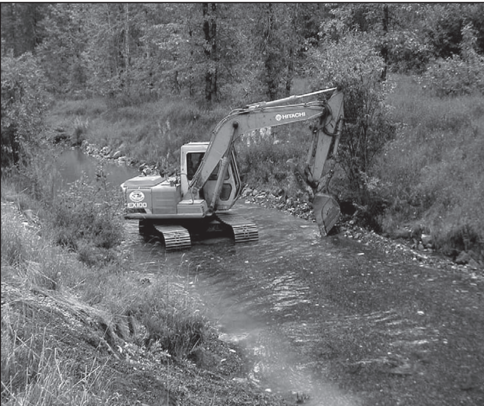
Turner Construction rebuilds the Herman Creek spawning channel 25 miles north of Haines
