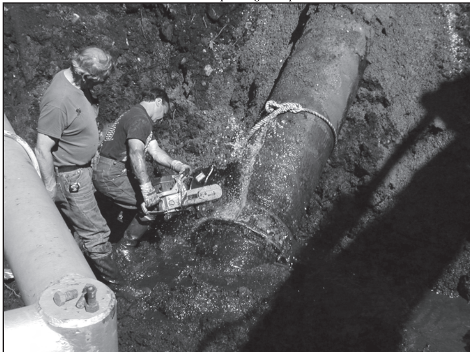
Conner Nelson and crew work on repairing the penstock at Hidden Falls.
