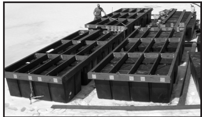
New project leader Josh Homer works on the construction of a feed float at Deer Lake.
