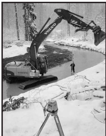
The new Herman Creek Spawning Channel was completed in late November.
