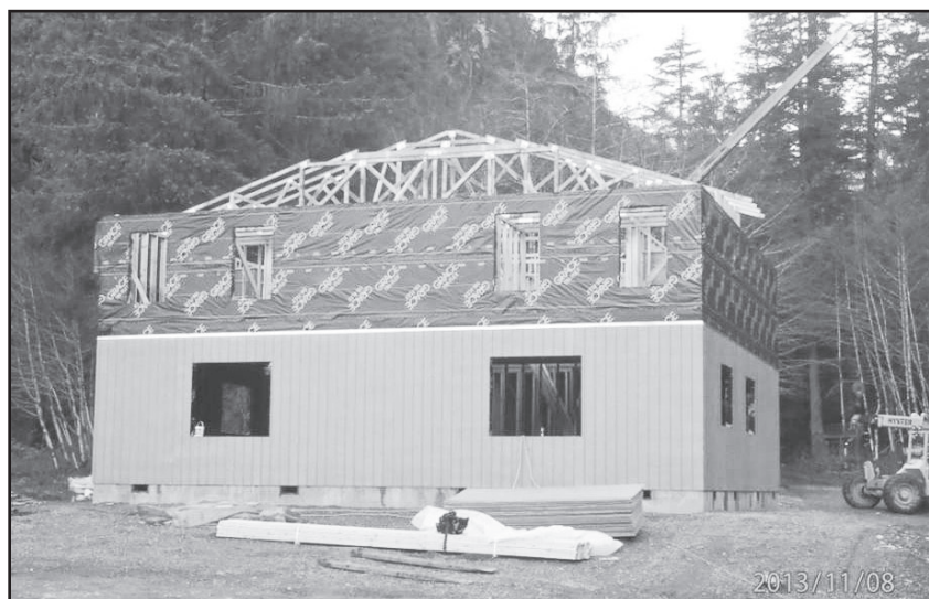
A duplex is currently being constructed at Medvejie. This will be a great improvement to housing needs at the hatchery.
