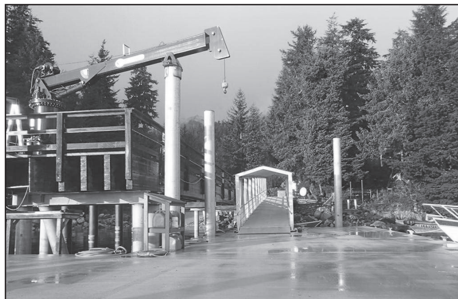
Hidden Falls’s new dock is a reality. Construction took place this summer.
