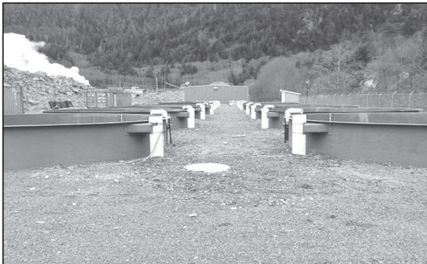
Round pond complex at Sawmill Creek. Over 1 million coho will rear in these ponds in 2014.
