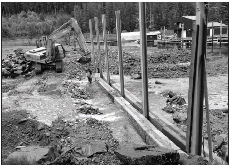
A new weir was installed at Medvejie this summer. It is a major improvement from the old structure.
