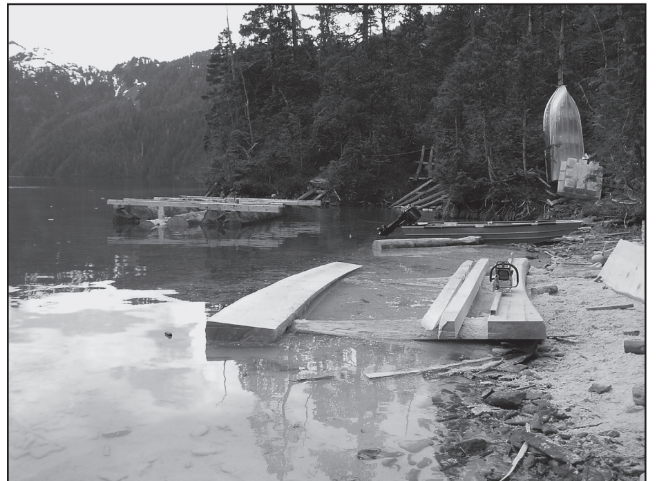
Timber in the process of being sawn for a feed storage float at Deer Lake.
