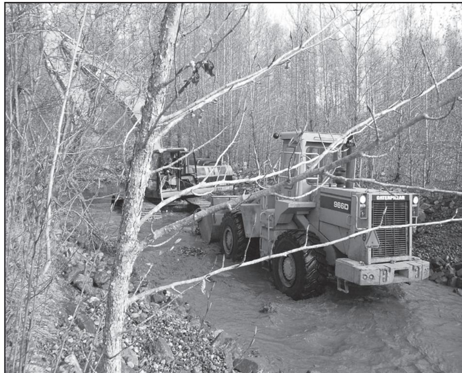
Construction crews work to replace gravel at 24 mile spawning channel in Haines this spring.
