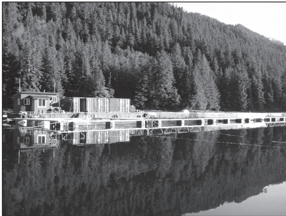
A view of the barge and net pen complex at Deep Inlet this spring.
