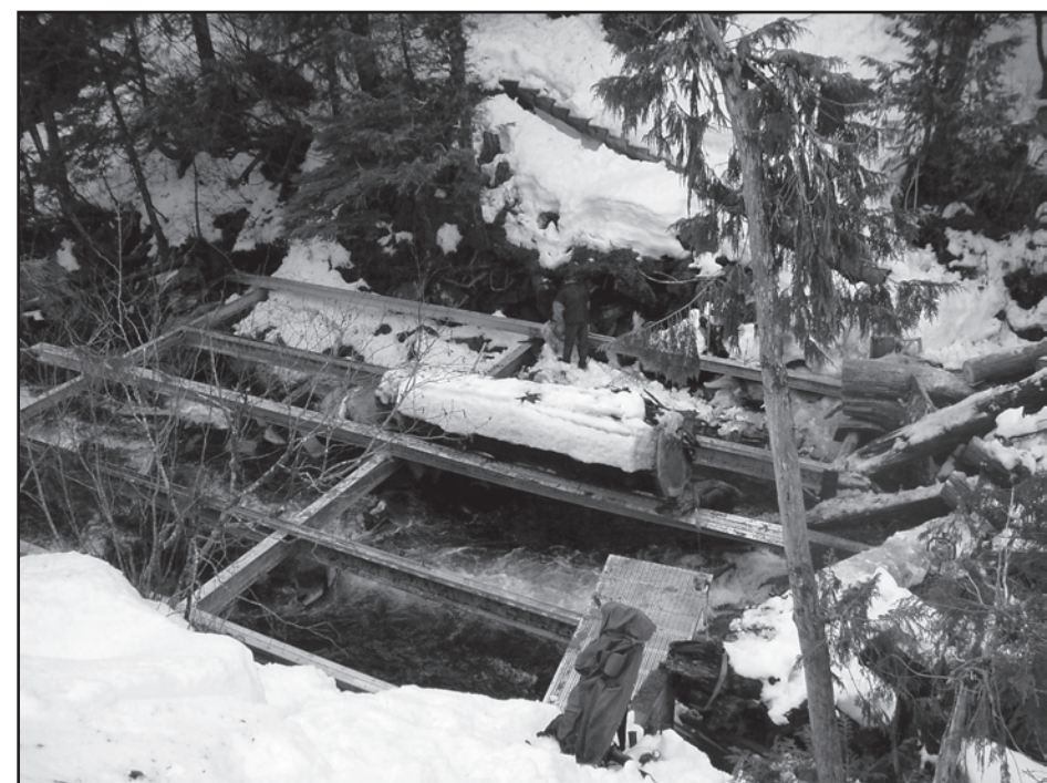
Josh Homer works to clear the Deer Lake weir after the high water event.
