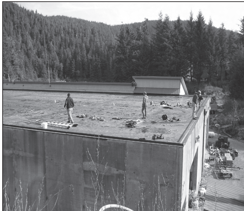
Coogan Construction works on replacing the roof of the incubation building at Hidden falls this spring.
