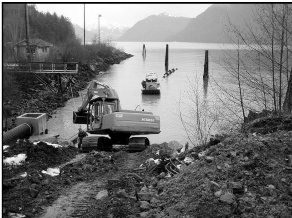
Keystone Construction workers set the effluent pipeline for the Sawmill Cove Hatchery.
