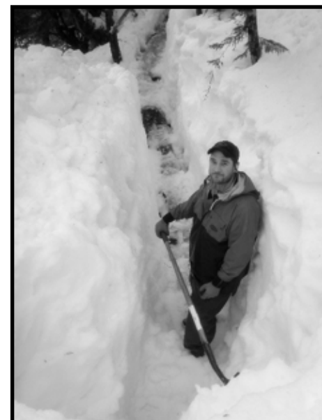
Josh Homer clears the smolt pipeline route at Deer Lake. Josh will take over as project leader July 1, 2008.
