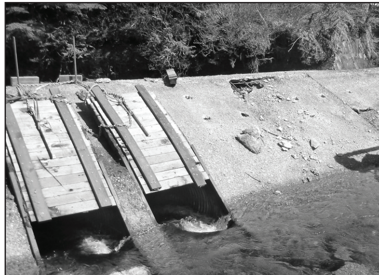
Hidden Falls staff discovered a gap in the dam this spring. The hole can be seen on the dam face in the middle right side of this photo.
