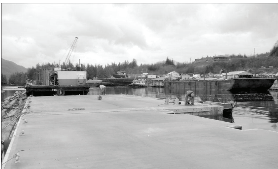
The deck of Hidden Fall's new dock was fabricated in Prince Rupert and was towed to the hatchery in April.
