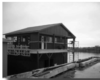
PR Concrete Floats of Powell River, B.C. is finishing construction of a new barge for Deep Inlet. The barge will provide housing and feed storage for spring rearing and is scheduled to be delivered in time for the 2010 rearing season. Clockwise from upper left: pouring the concrete deck, finishing the deck, framing, finishing the living quarters.
