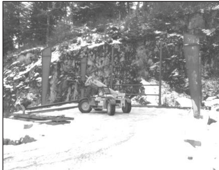
Work is underway on a new 50' x 50' incubator storage building at Hidden Falls Hatchery. The building will house the extra incubators needed for the Southeast Cove chum project when they aren't in use at the hatchery.
