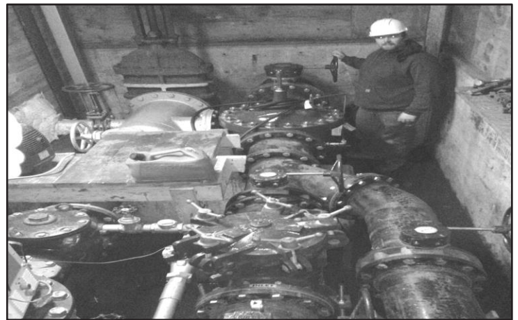
Maintenance Engineer Kenny Gray adjusts a valve on the new PRV (Pressure-Relief Valve), a critical part of the water supply to Sawmill Creek.
