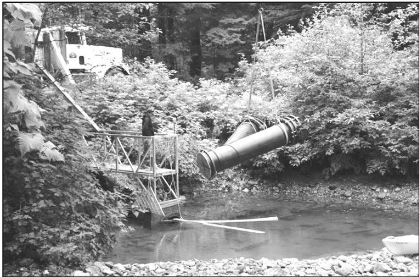
Major improvements were completed on Medvejie's water supply system this summer. Above: A new intake is lowered into position.
