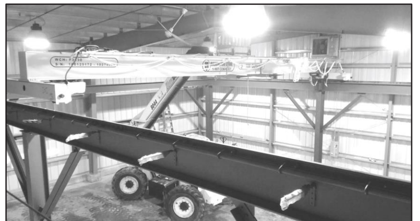
Mike Pountney positions Sawmill Creek's bridge crane into place. The crane is used to empty incubators.
