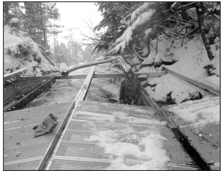
Woody Cyr, project leader at Deer Lake, installs weir panels this past spring. The weir funnels emigrating smolts into a pipeline which transports them to saltwater net pens, bypassing the lake's 300 foot waterfall.
