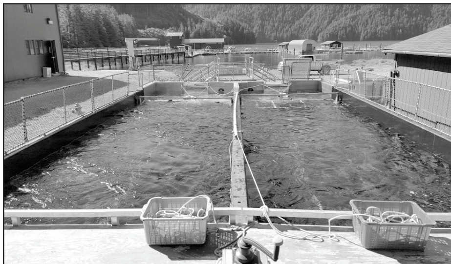
Aluminum raceway extensions provide more holding capacity for chum spawning at Medvejie. This improvement should allow staff to process more fish each day and increase the efficiency of egg-takes.
