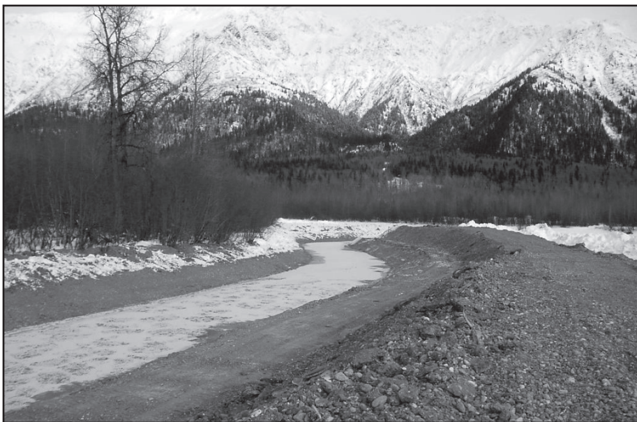
Phase I of NSRAA's new Confluence Spawning Channel was completed in March. Construction costs were covered by a state grant secured by Representative Bill Thomas.
