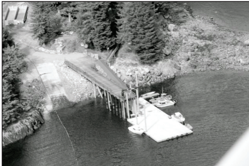
Hidden Falls dock and barge ramp are now complete.
