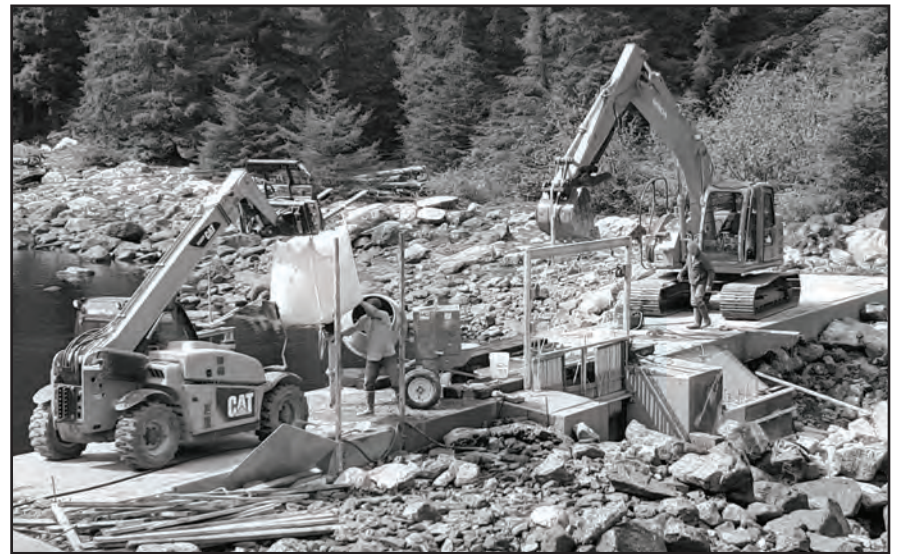
Keystone Construction employees work on the Hidden Falls weir this spring. Upgrades to the weir will improve broodstock management at the hatchery.
